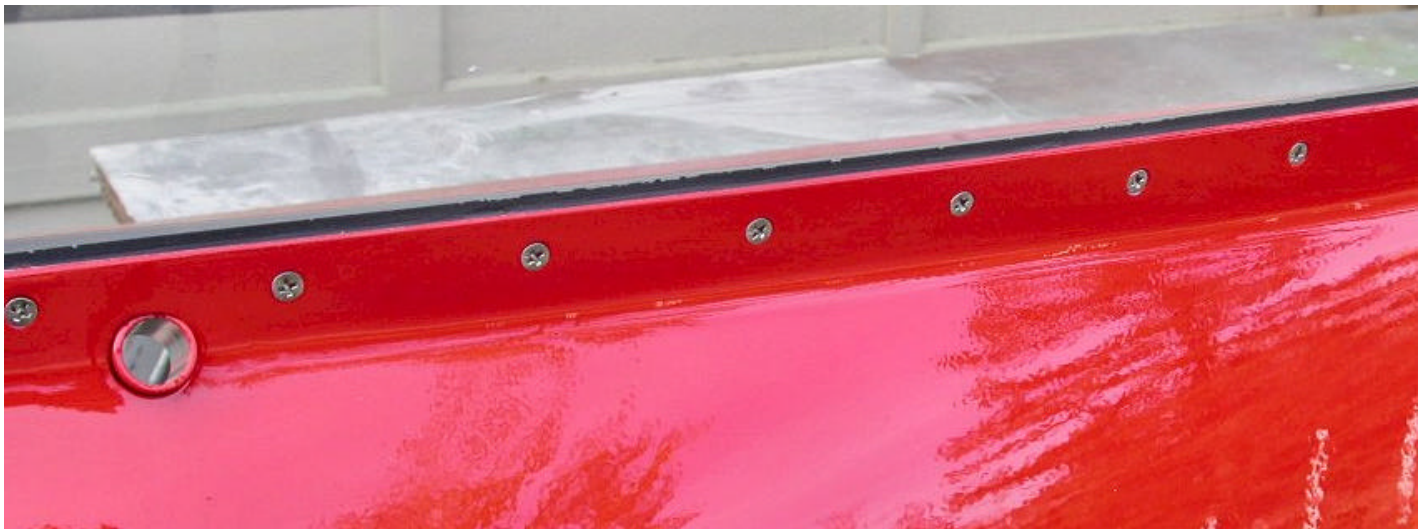
ABOVE: The finished installation with the stainless steel #6 screws clearly visible.
